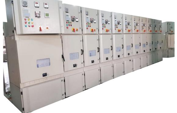
A VCB Panel is a types of circuit breaker where the arc quenching occurs is vacuum environment. VCB technology is ideal for medium voltage application .vacuum circuit breaker is renowned technology for medium voltage today and is also know as the most reliable current interruption technology for medium voltage switchgear.
